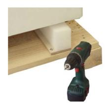
Screw the "Etafon" on the palette and then put the unit on.
