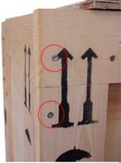
Screw in the screw heads flush. Don't counterbore the screws in the wood!
